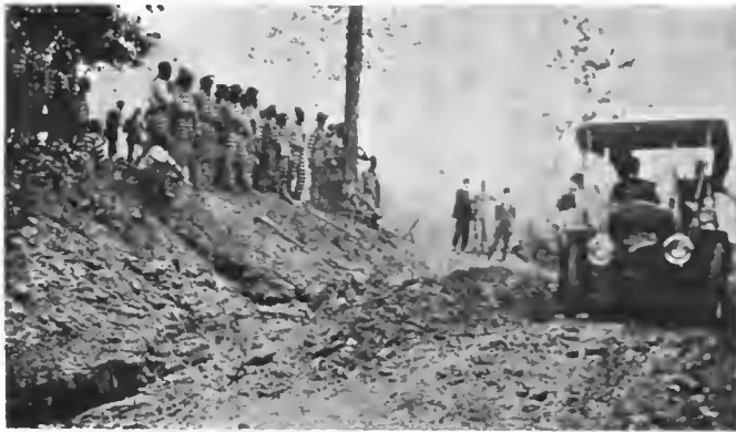
Georgia Convicts Cutting Road Through Solid Rock.
